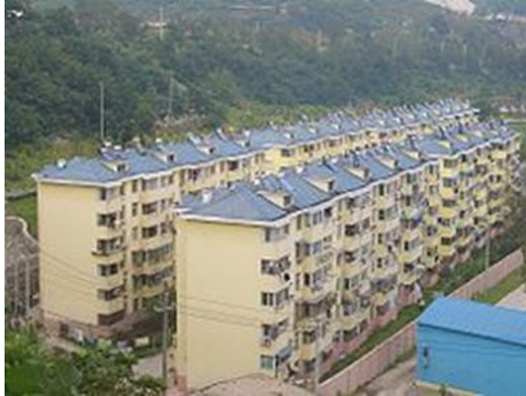
Solar power water heaters are very popular among middle sized cities in China.
