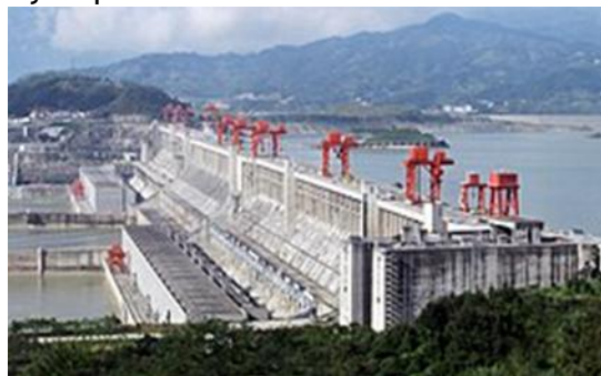
Three Gorges Dam hydroelectric power plant in Hubei, China
