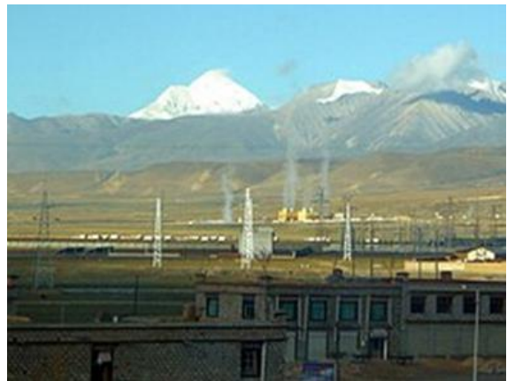
A 24 MW power station in Yangbajain Geothermal Field
