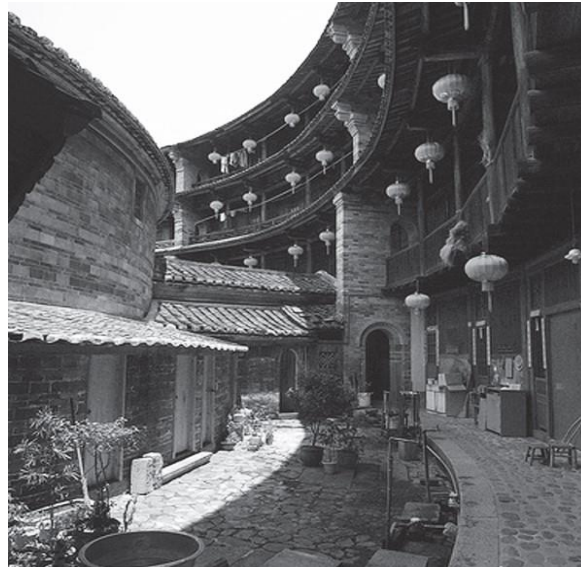
THIS IS A REPRESENTATIVE VIEW OF THE UPPER STRUCTURE OF A ROUNDHOUSE. NOTE THE UPPER FLOOR IS CANTILEVERED OVER THE LOWER AND THE USE OF MANY BAMBOO BASKETS.
