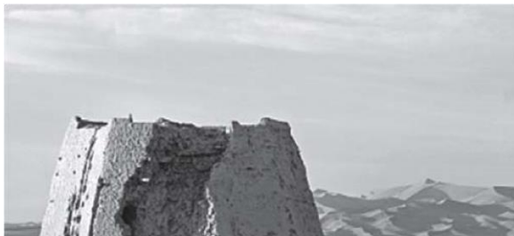
The ruins of a Han dynasty (202 BC – 220 AD) Chinese watchtower made of rammed earth, Gansu province. Part of Emperor Wu's extension of Han's defence lines to the western regions.
